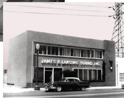
James B. Lansing and early headquarters facilities of JBL in Southern California..
