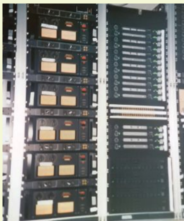
The processing and amplifiers for the system at Orchard Hall in Tokyo, Japan in 1988 or so. This system had an abundance of subdivision: left/right, upper/lower, inner/outer, and so on. The amplifiers are in the left rack, and single channel loudspeaker processors are in the rack on the right.
