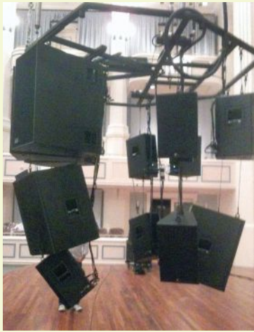
A highly subdivided center cluster in a symphony hall with extremely complex 360-degree seating (and only one hang point). The front mains have upper/middle/lower subsystems with inner/outer. There are three subsystems for the sides and another for the rear. A total of nine channels of signal processing (EQ, level and delay) were needed. Each cabinet has independent pan and tilt to help facilitate optimal vertical and horizontal aim and splay.
