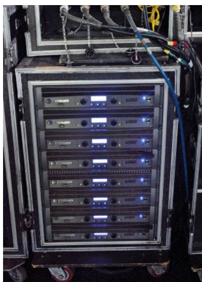
A rack of Crown I-Tech 12000HD amplifiers. The tour carries more than 40 to drive all loudspeakers in the full rig.
